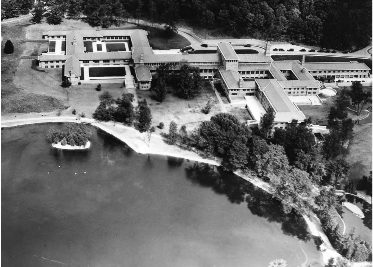
Figure 2.21 The nearly completed Kingswood School complex occupies the northeast shore of Kingswood Lake directly north of the Japanese Garden in 1931. The construction of the school results in changes to the waterways, character of the shoreline, features of the islands, and types of vegetation in the garden.
