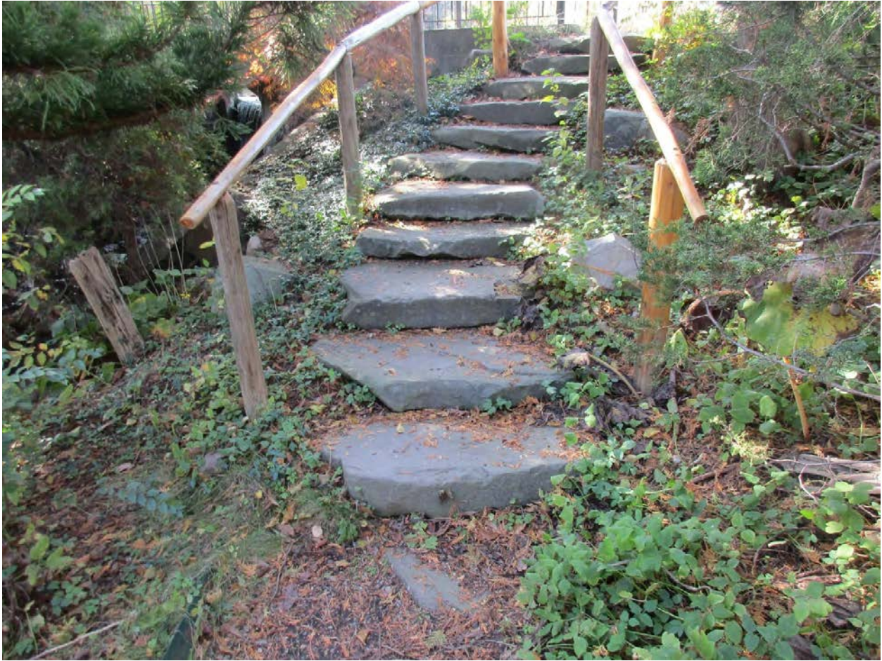
Figure 3.36 Stone steps between the Lakeside Walk and the lower west walk. An older fence post projects from the slope to the side of the new railings. QEA, October 2017.
