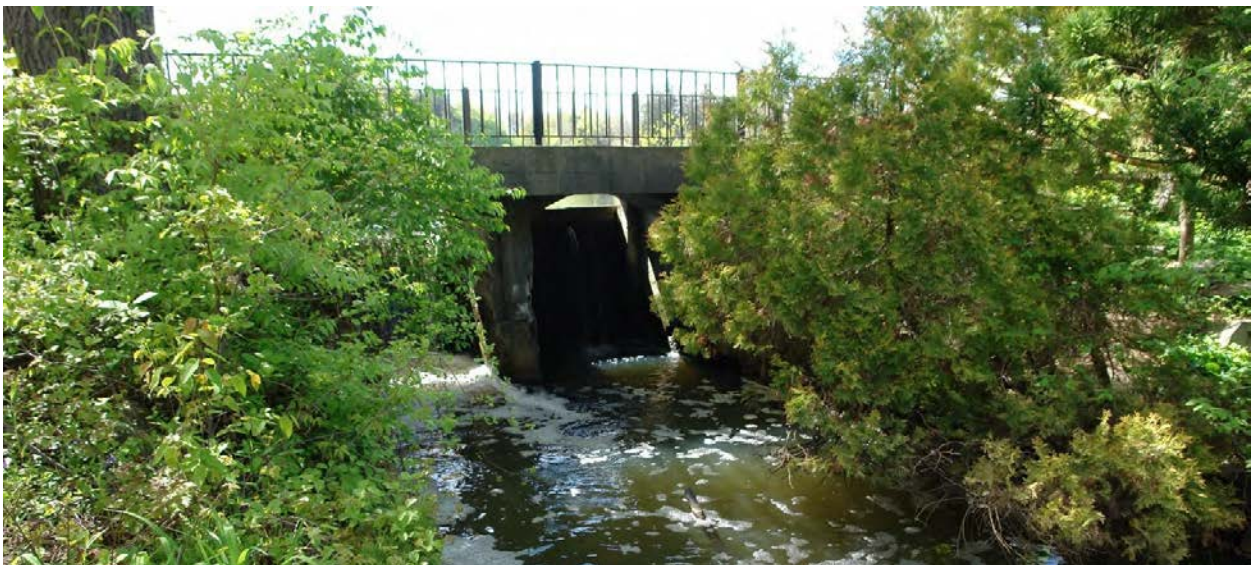
Figure 3.37 The bridge at the East Water Gate on the Lakeside Walk spans the inlet for the Lily Pond. QEA, May 2017.
