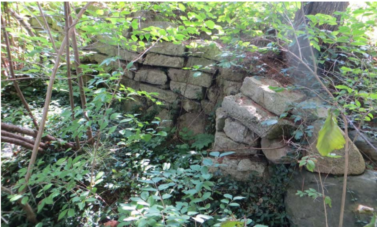
Figure 3.42 Stacked concrete blocks form a retaining wall below the Lakeside Walk north of the East Water Gate. QEA, August 2017.
