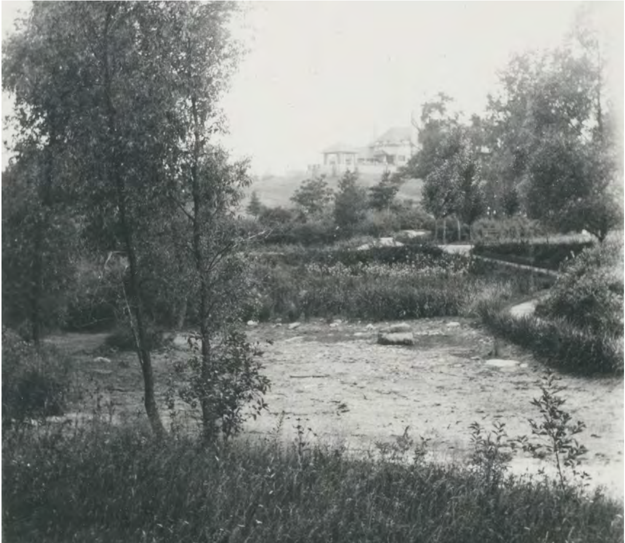
Figure 2.3 View southwest showing a dry water body, paths, and recent plantings in the Japanese Garden area, ca. 1909.
